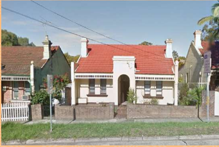
BEFORE: The historic cottage at 77 Old Canterbury Rd, Lewisham
