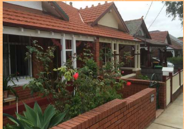
Beach Rd single fronted Federation style cottages
