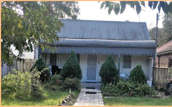
Weatherboard house in The Parade
